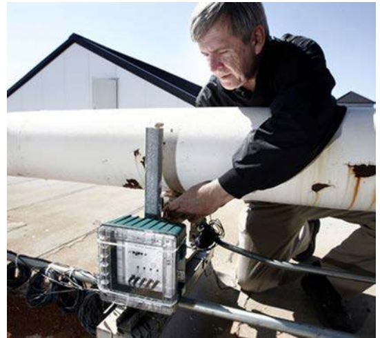
Pest control operator installing the Ultrason X, an ultrasonic bird control device.
